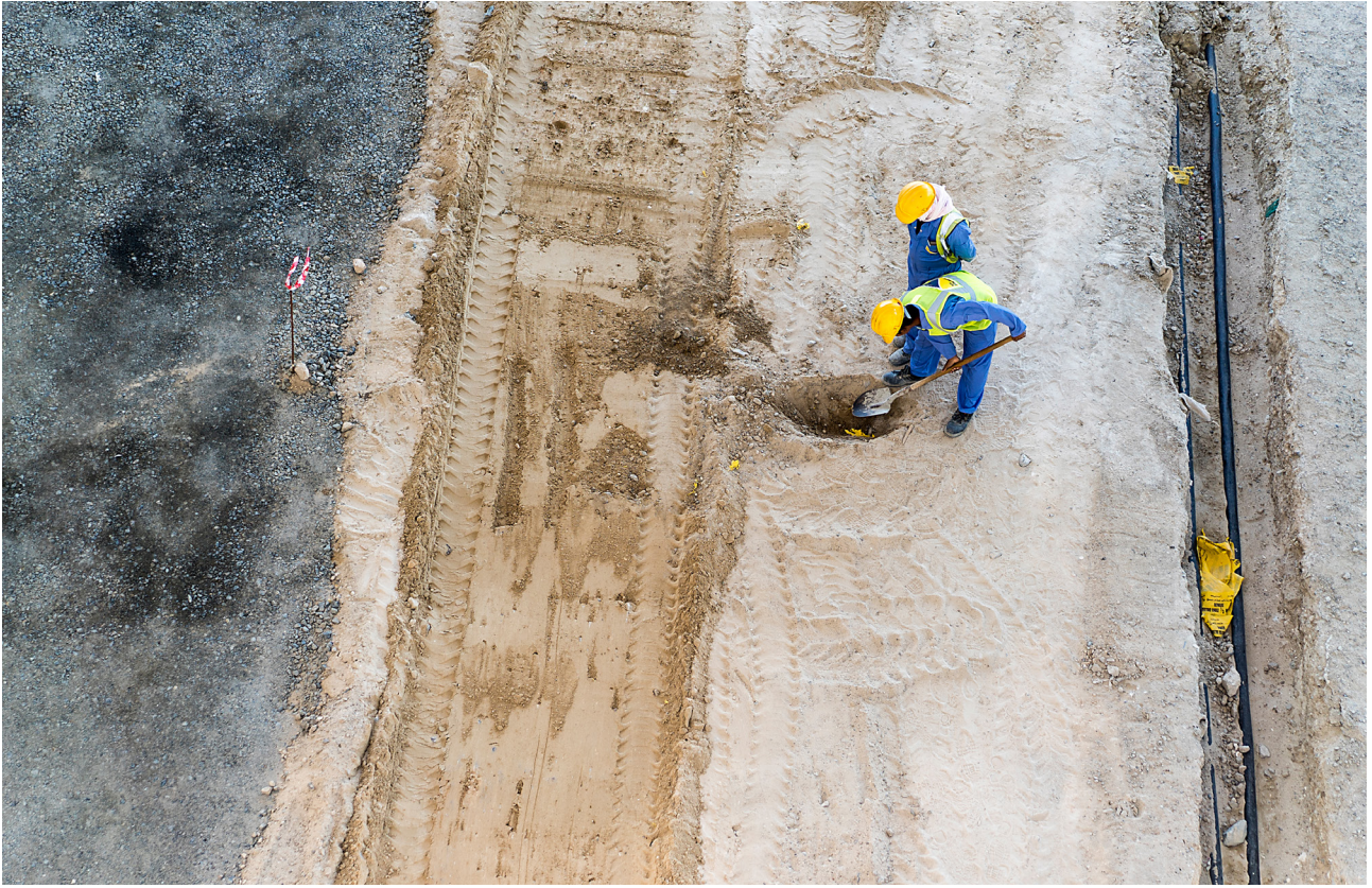
Construction Workers, Dubai
